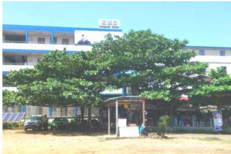
Keeping the KMD Institute training premises clean and green
