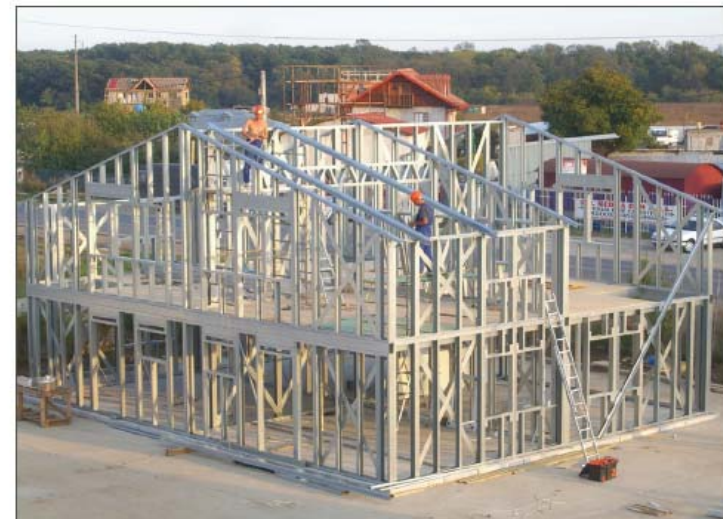
ArcelorMittal steel frame house for Habitat for Humanity
